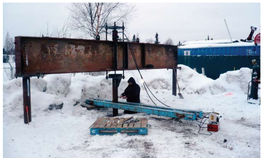
AXIAL TENSION (UPLIFT) LOAD TEST SETUP
