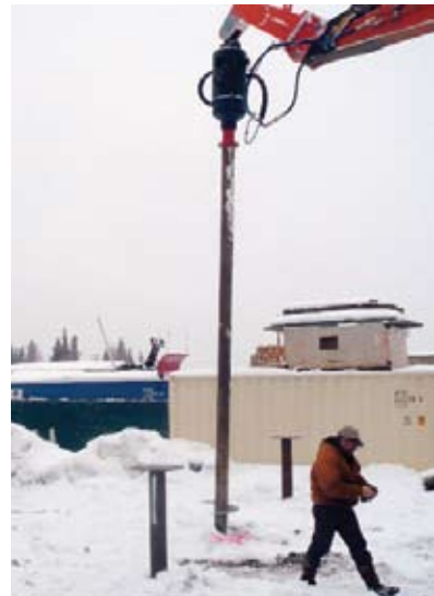
TYPICAL HELICAL PILE INSTALLATION
