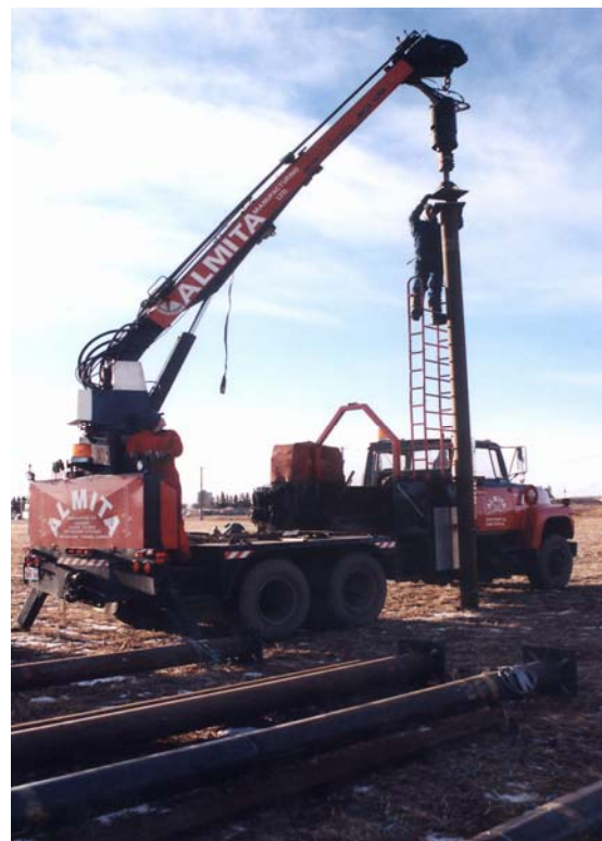
Figure 2. Screw Anchor Pile Installation
