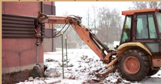
Underpinning application of helical foundations.
