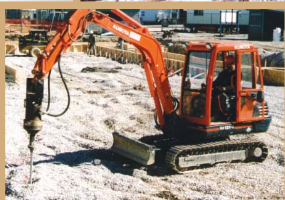
Installing helical foundations for structural slab support.
